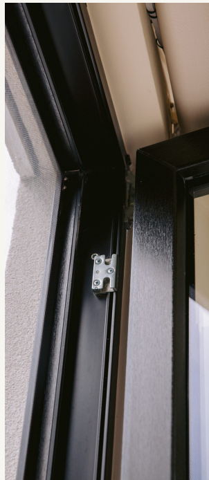
CONCEALED LOCKING POINT, TILT-TURN
